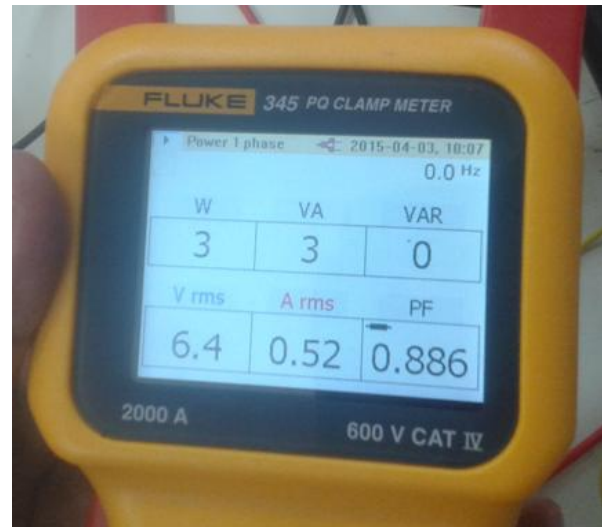
Fig.17 Power Factor of the Supply Current measured by PQ Analyzer
