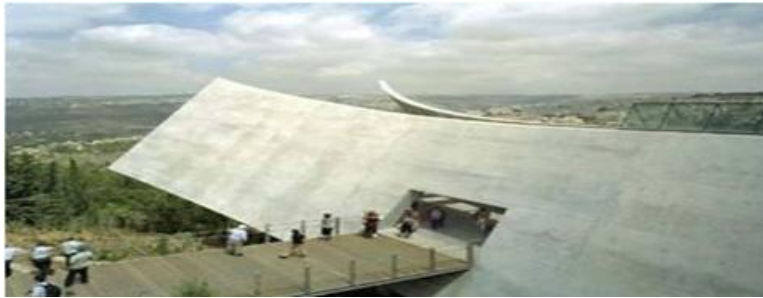
Fig. 13. Main entrance of the building
