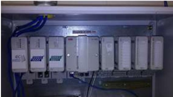
**Figure 4 (a)** ABB 800 XA with interfacing of devices that support multiple protocol
