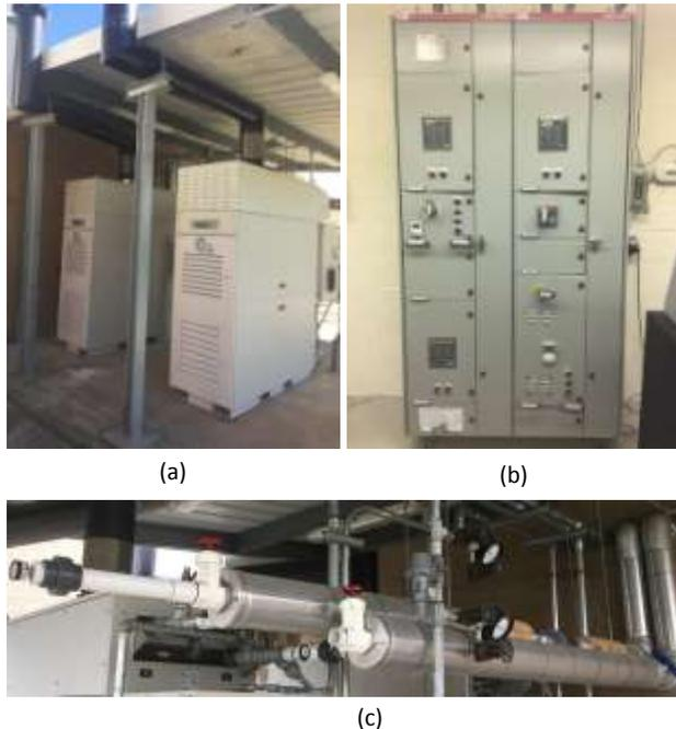
**Figure 2.** Photograph of Microgrid Equipment (a) two Capstone micro turbines (b) Machine Control Center (MCC) from ABB Inc. and (c) water inlet-outlet piping to recapture unused heat
